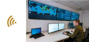
Brunvoll Operation Centre - for remote access & assistance
